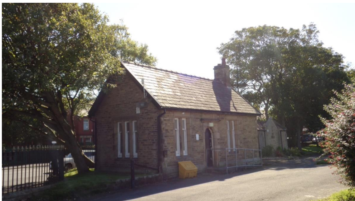
Locally listed lodge now used as an office
