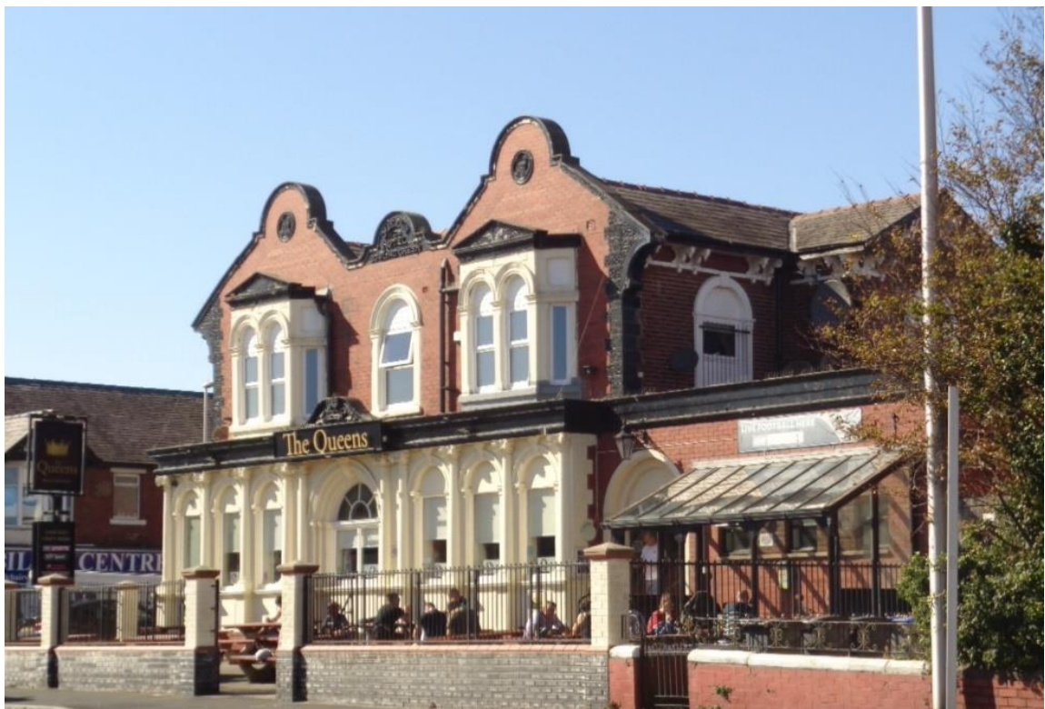
Queens Hotel, Talbot Road
