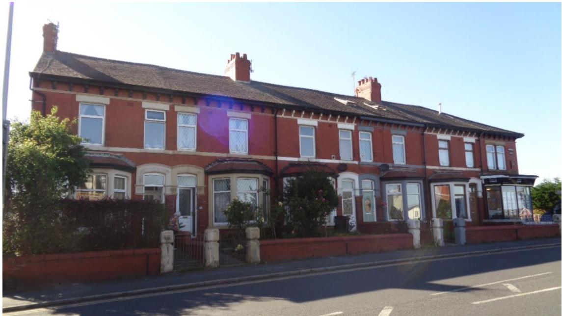
Edwardian terrace with single storey canted bays to the north of St. Mark's parish church
