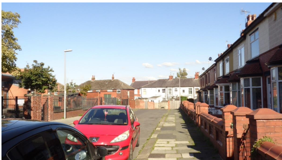
View of rear of properties on Melrose Avenue at the north end
