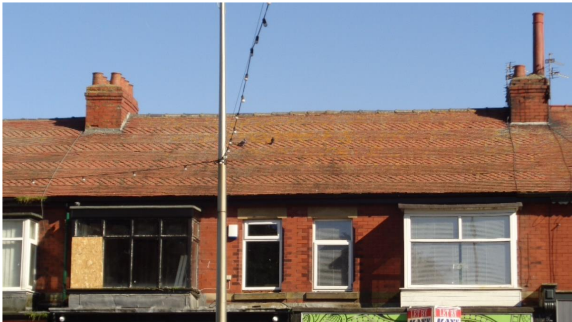
Decorative red clay tile roof covering to 1 – 21 Layton Road
