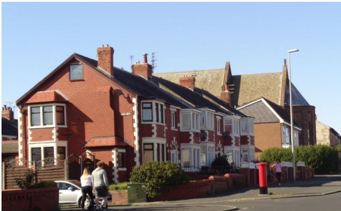
Interwar housing on the site of Layton Villa gardens
