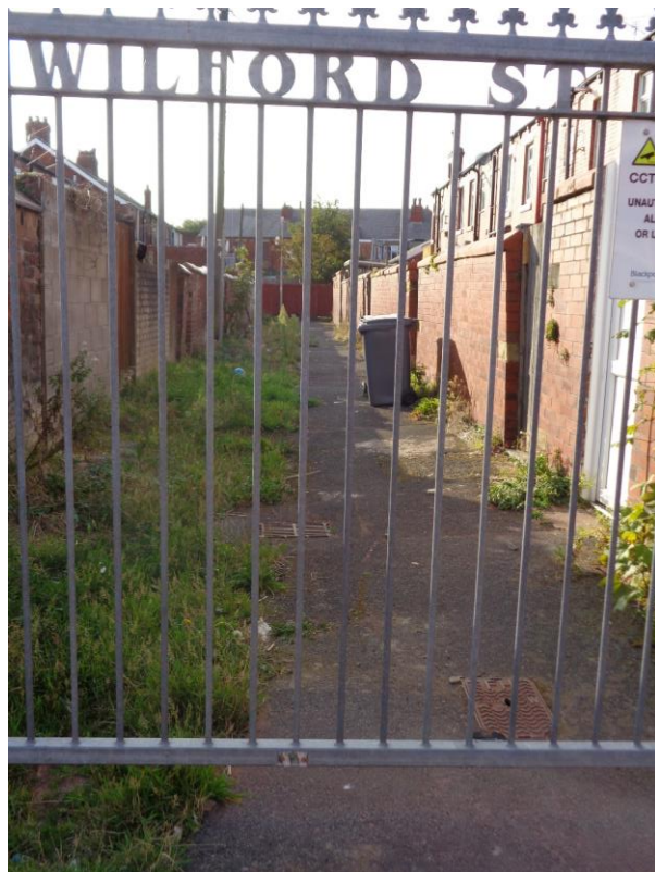
Alleygate on Wilford Street
