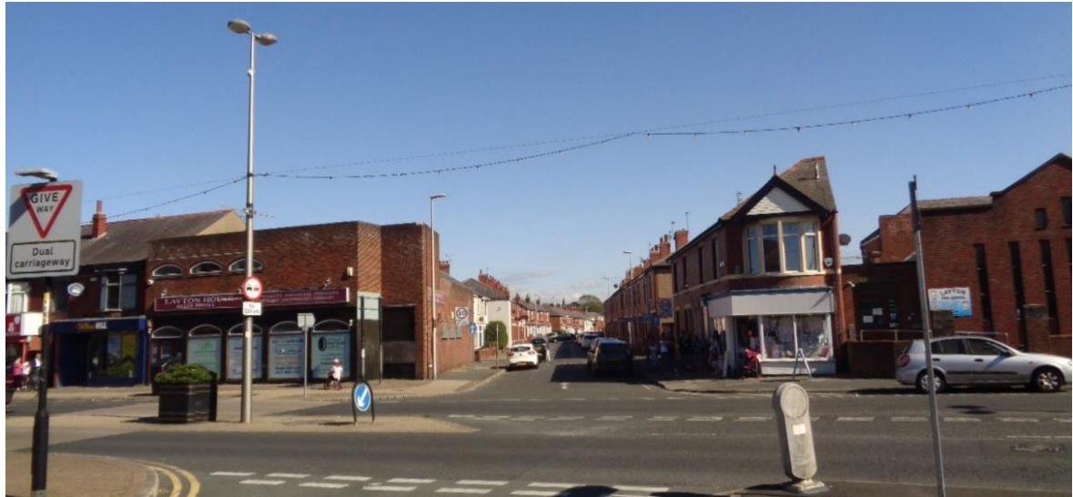
View east down Grenfell Avenue from the junction of Annesley Avenue/Westcliffe Drive
