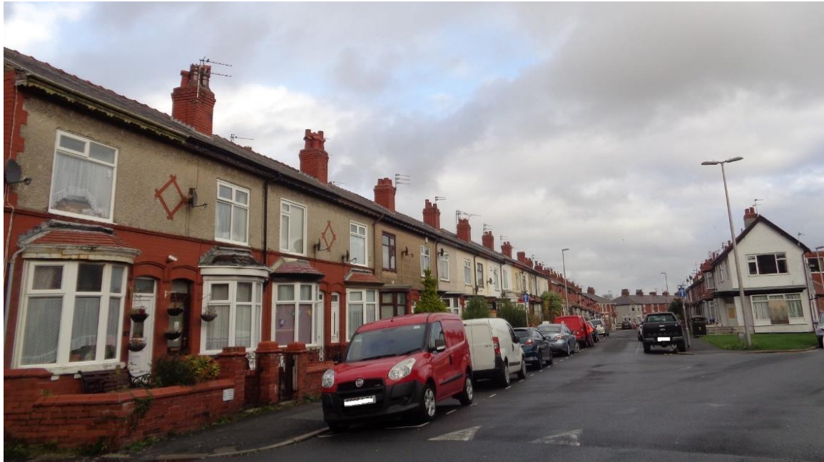
1 – 31 Onslow Road view views of the side elevation of 28 Onslow Road
