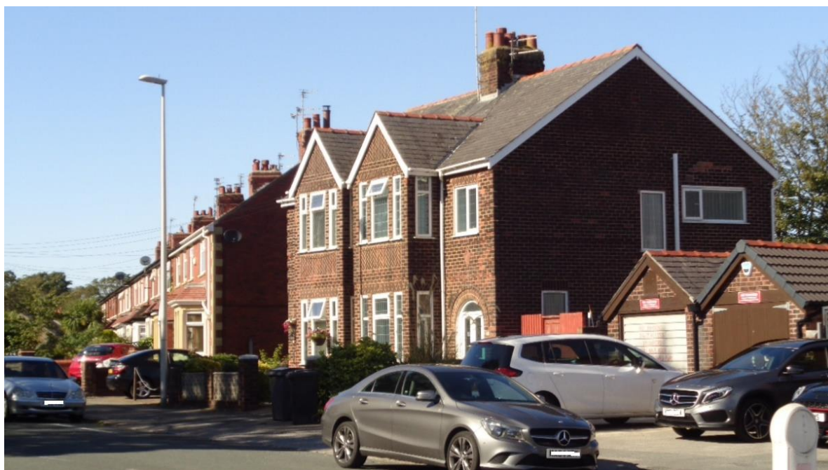
Numbers 2 – 4 Annesley Avenue looking west
