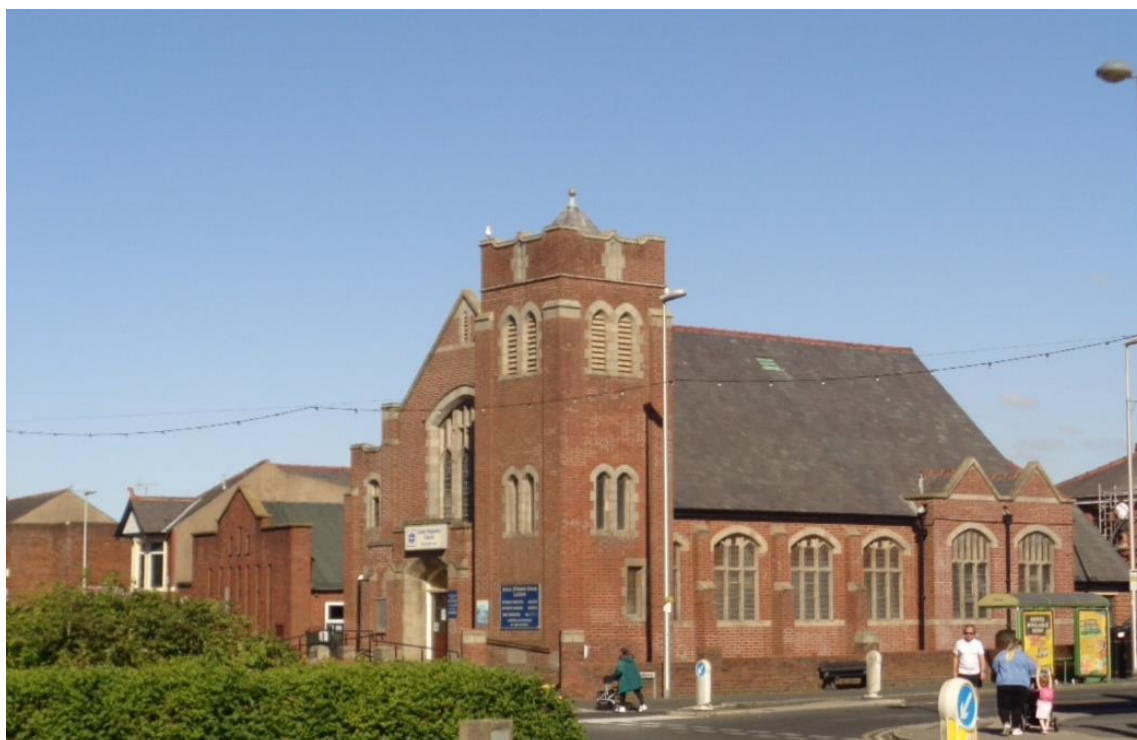
Locally listed Salem Layton Methodist Church with adjacent church hall
