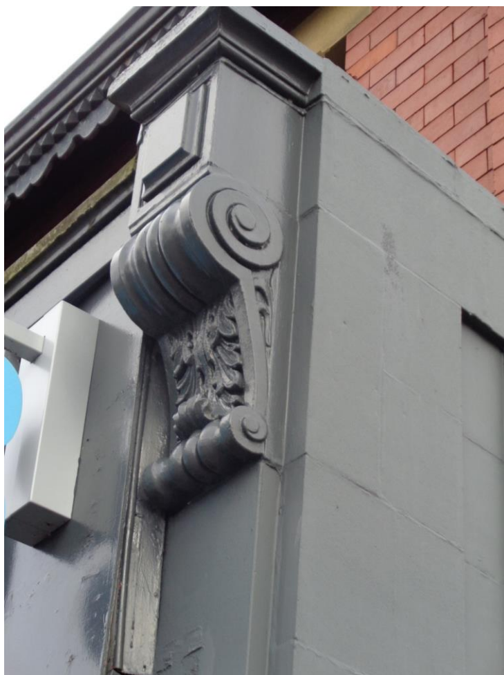
Console bracket on Co-op frontage
