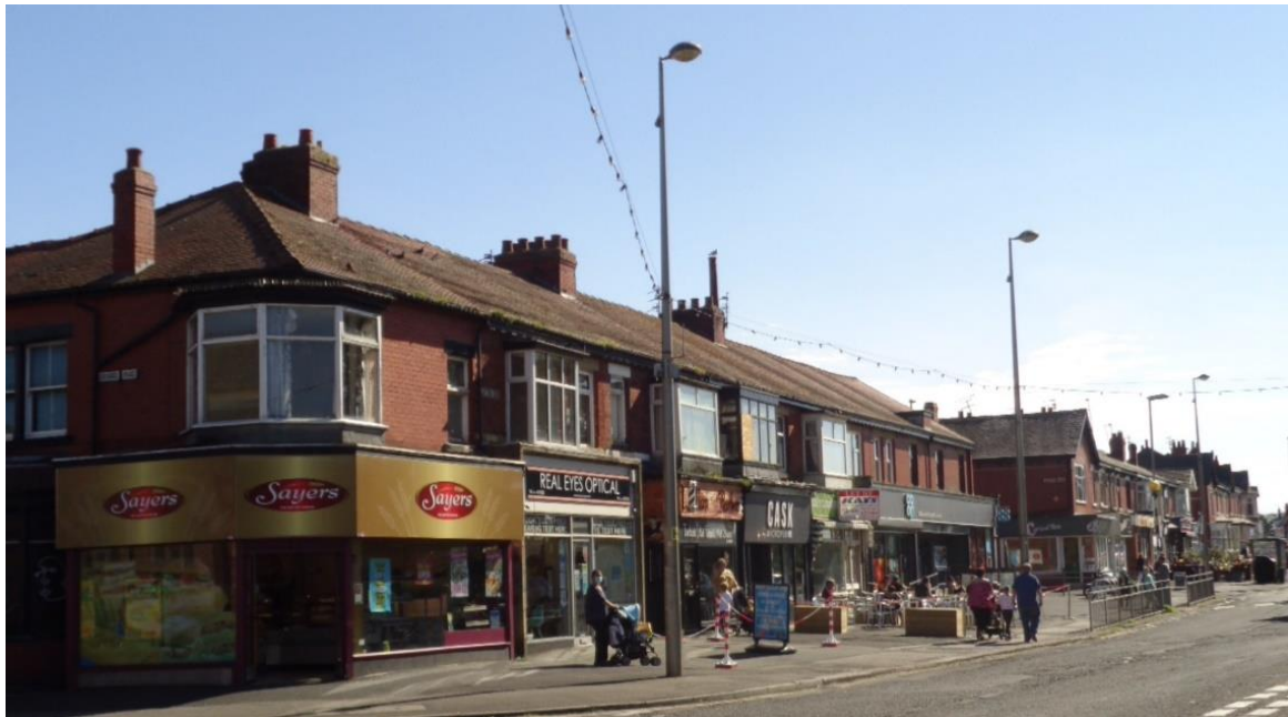
Numbers 1 – 21 Layton Road viewed from opposite the Grange Road junction
