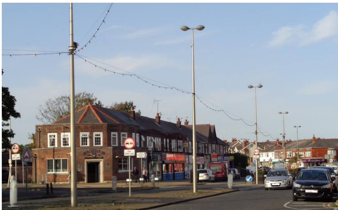
Purpose built shops 2 – 28 Westcliffe Drive
